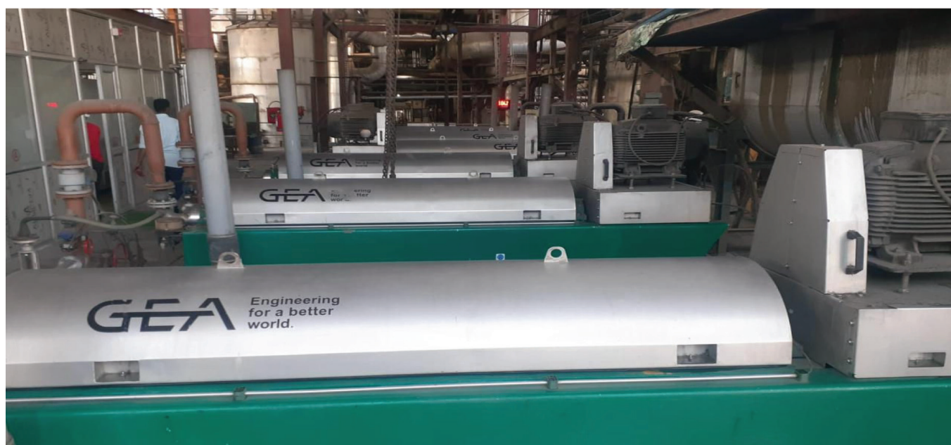
Figure 8 : Installation of decanters at SSM
