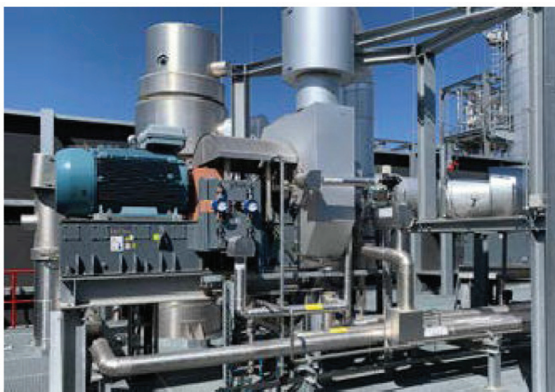
Figure 3 : PLLER High - Performance blower in the bio-ethanol plant
